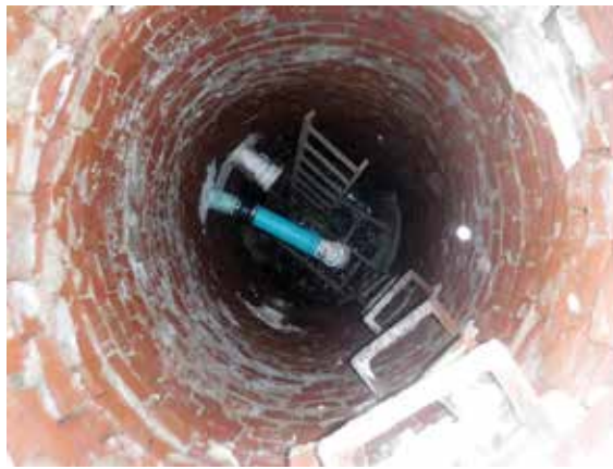
Water ran against the bricks of this manhole, which is more than 80 years old, causing it to lose mortar and some of its bricks. Infiltration from a broken stormwater pipe nearby then made its way into the sanitary sewer system.
