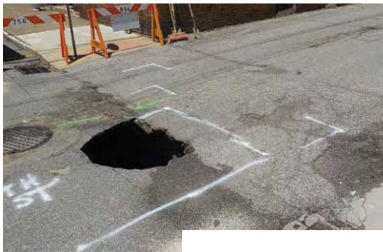
A garbage truck fell into a sinkhole next to a manhole that had eroded and deteriorated due to infiltration from a broken stormwater drainpipe nearby.
