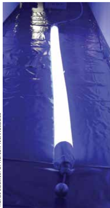
Curing doesn’t begin until the light train inside the liner is activated, which allows for more time to assure a quality installation.
