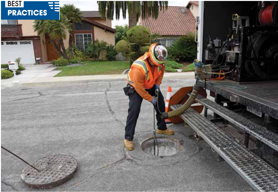
Camera systems using lateral launch technology have made a big impact on cross-bore detection.
