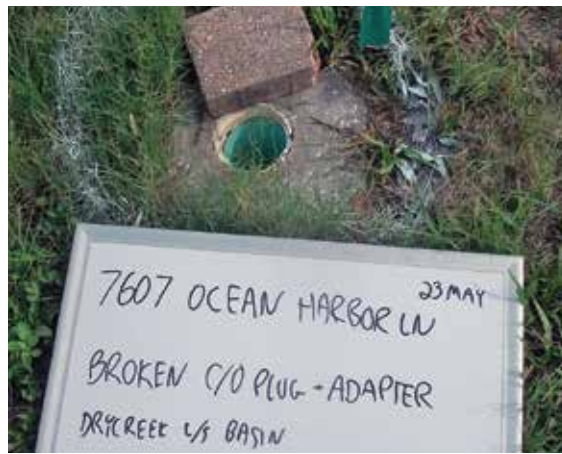
Crews use whiteboard notes and paint to mark sources of I&I discovered via smoke testing. Here, a broken cleanout plug (left) and an electrical utility box (right) are marked for repair.
