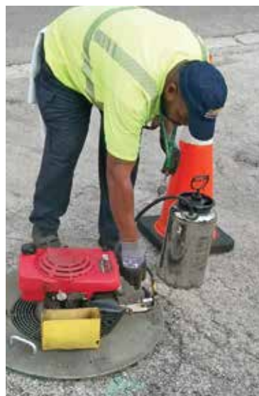
A worker sets up smoke testing equipment at a manhole.
