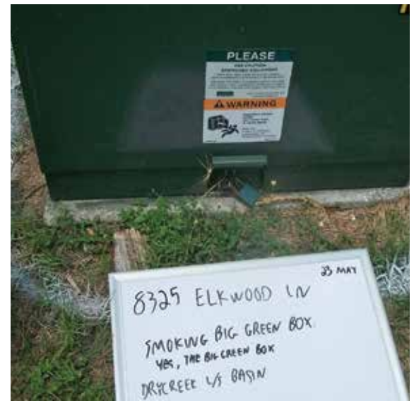
Crews use whiteboard notes and paint to mark sources of I&I discovered via smoke testing. Here, a broken cleanout plug (left) and an electrical utility box (right) are marked for repair.
