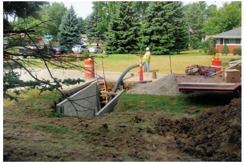
The district is exploring the use of more invasive lateral repair techniques in some cases, including pipe bursting.
