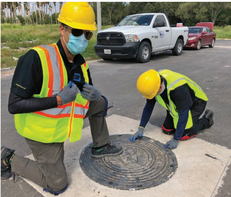
A finished composite manhole cover offers a watertight solution in the fight against stormwater infiltration.
