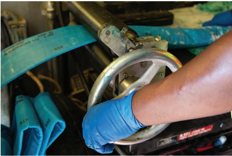
Preparing a CIPP liner with resin on a wet-out table.
