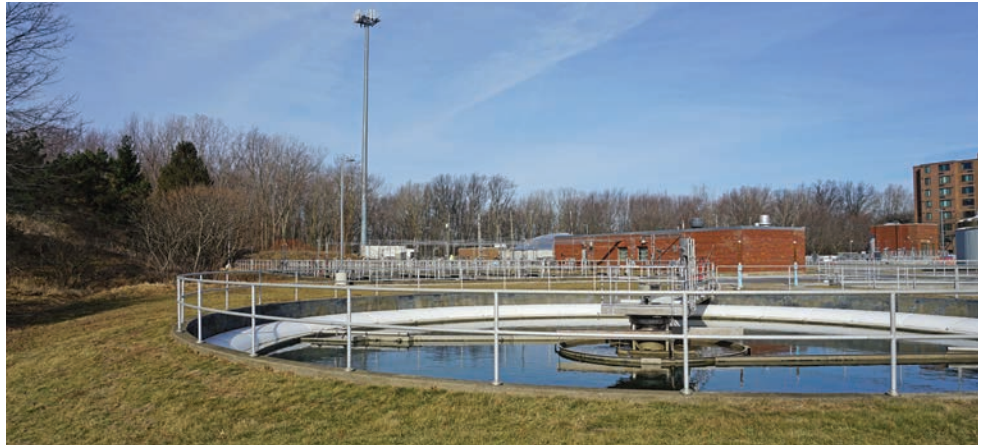
Avon Lake (Ohio) Regional Water's water reclamation facility provides the community's need for safe wastewater treatment. It has a capacity of 6.5 mgd and can accept flows as high as 12.5 mgd during wet-weather periods.
