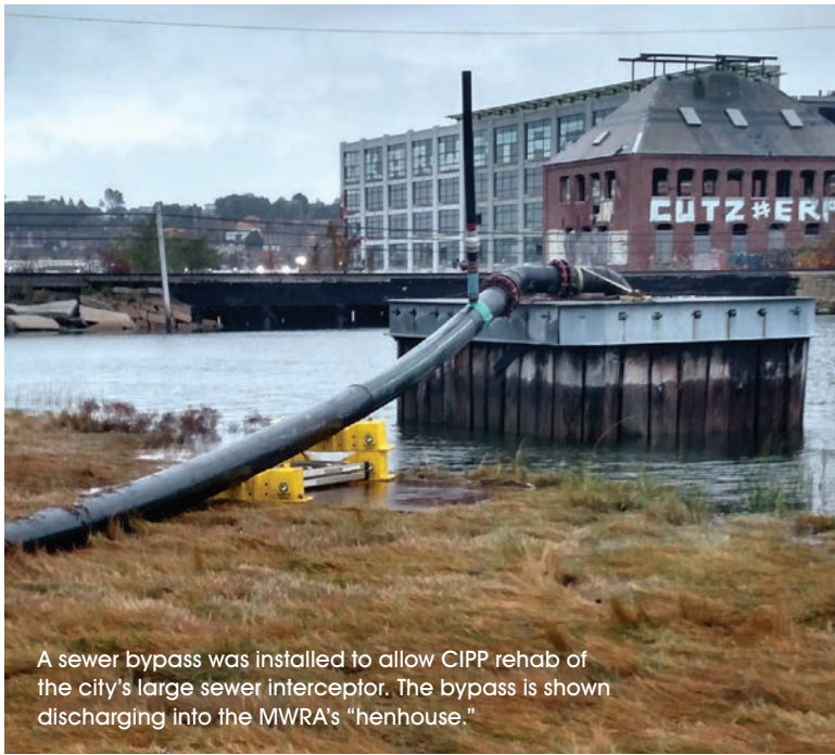
PHOTO COURTESY OF REVERE WATER AND SEWER DEPARTMENT
