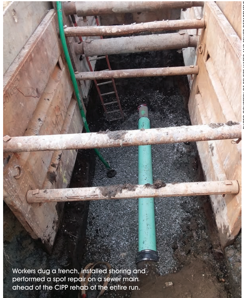
PHOTO COURTESY OF REVERE WATER AND SEWER DEPARTMENT
