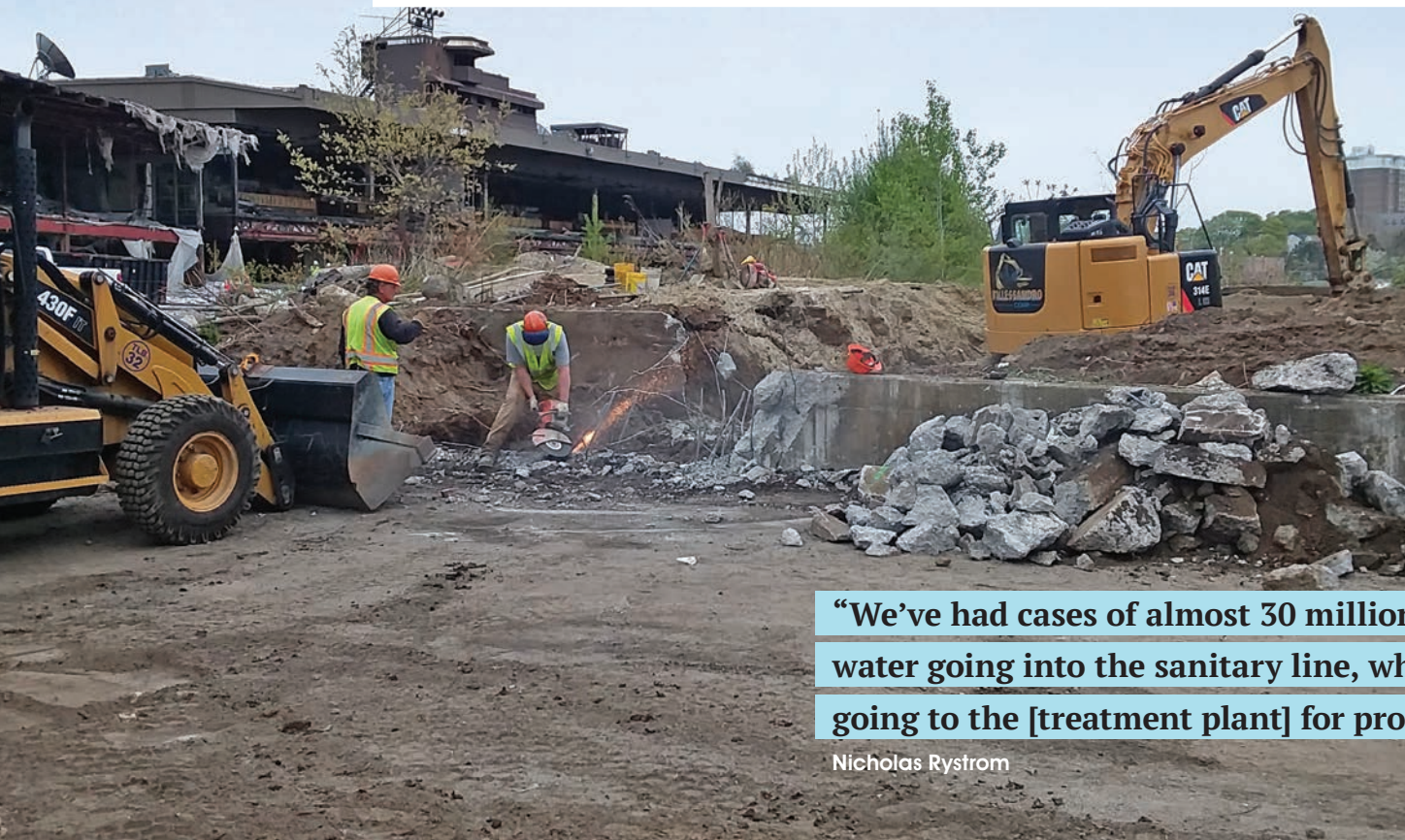
PHOTO COURTESY OF REVERE WATER AND SEWER DEPARTMENT
