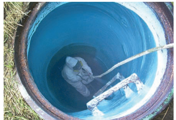
Manhole walls are sprayed to seal out I&I.
