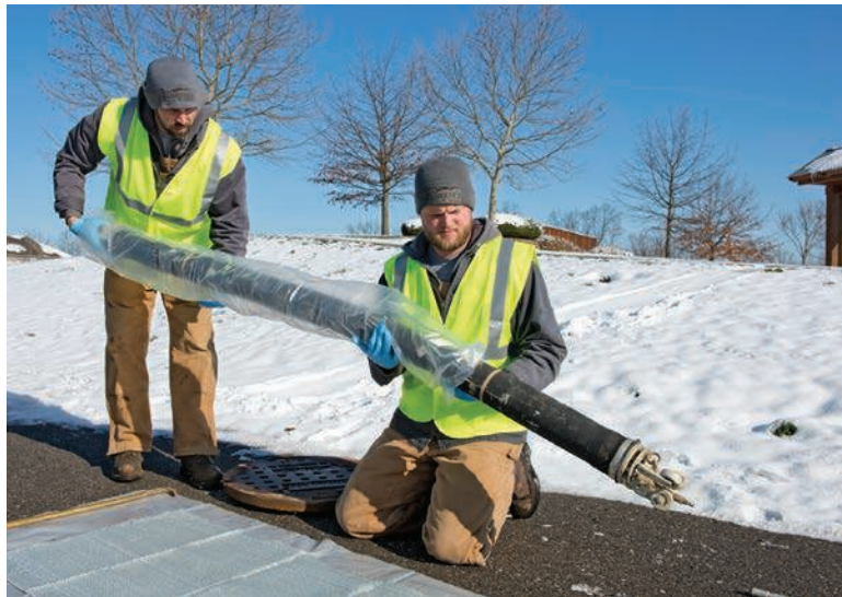
Maintenance workers Jeremy Gruelle (left) and Bryce Meier prepare a pipe patch for a sewer line repair.
