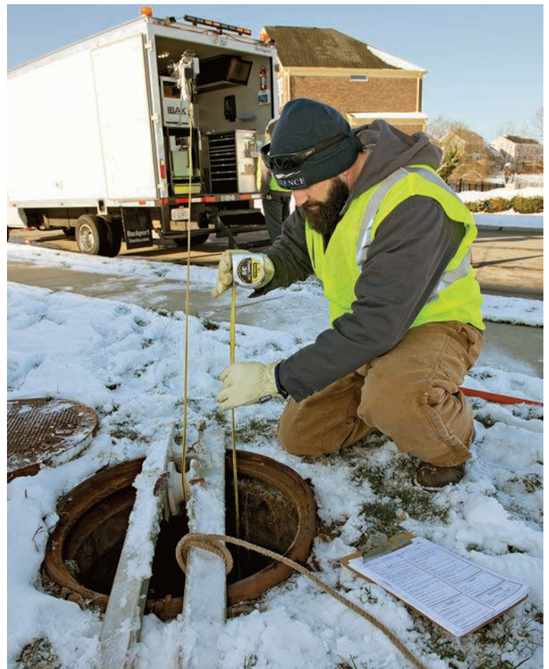
Florence Public Services Department maintenance worker Mark Teremi takes a depth measurement of a storm sewer.
