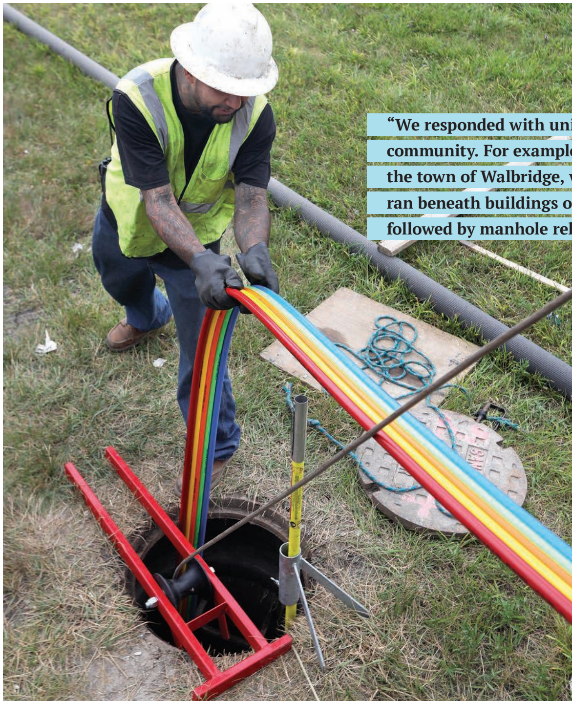
Anthony Velez pulls the grouting lines from the truck and guides them down a manhole during a rehabilitation project.
