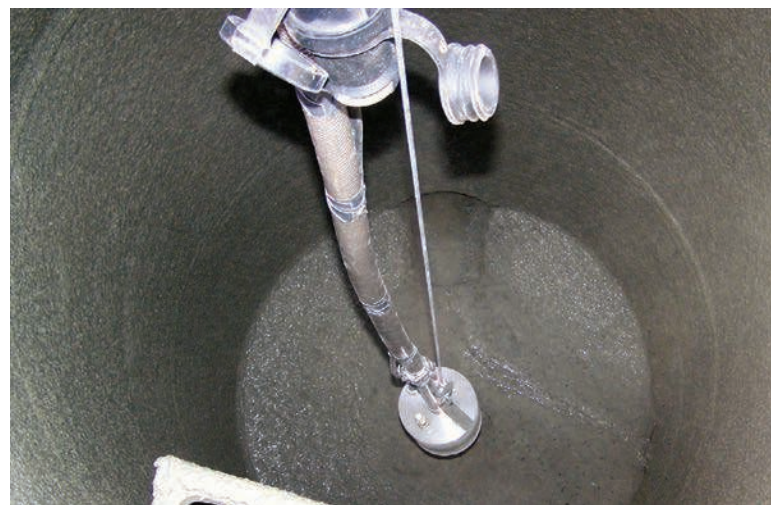
The Permacast system uses a bidirectional spin-caster that is lowered into the manhole and withdrawn vertically, so crews are usually able to avoid confined-space entry. The bidirectional motion eliminates concrete shadows caused by uneven bricks or other protrusions.
