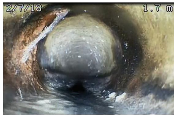
North Vancouver's push camera inspections of private-side laterals revealed cross connections (left) and infiltration (right) in many instances.
