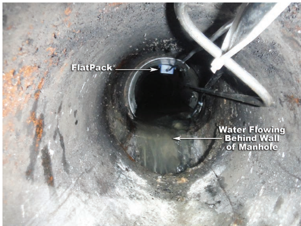
A view inside pipe A from the manhole, showing the FlatPack mounted at the top of the pipe.
