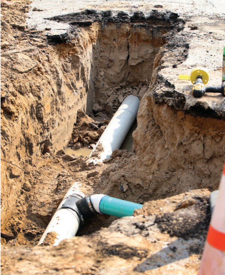
Pipe bursting helps Lufkin limit excavation to entry and exit pits and connection points.
