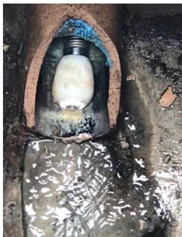
A push camera moves through a broken lateral line.
