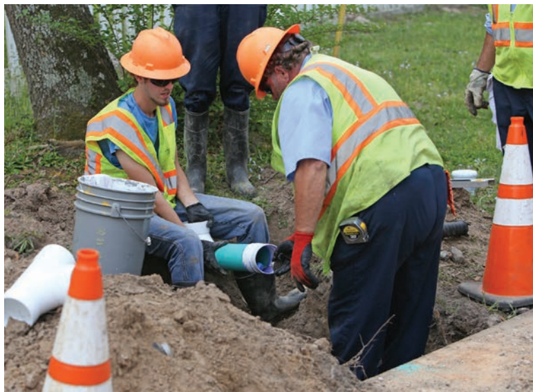
ABOVE: Crew members glue a fitting on a residential lateral connection after installing a new main. RIGHT: The main winch with the bursting head emerging below.
