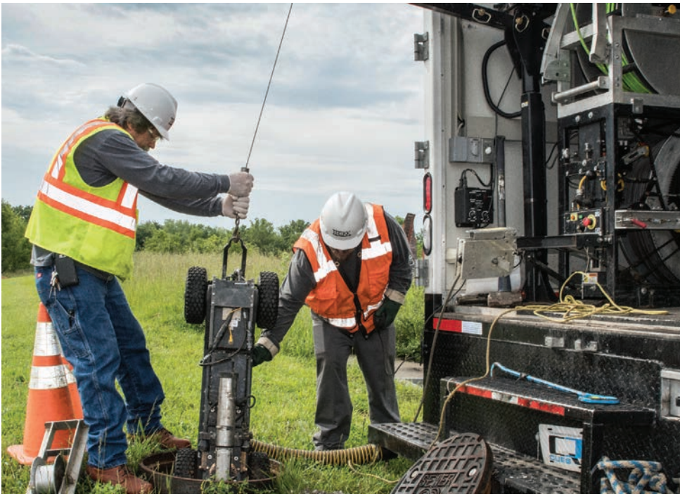
LEFT: An inspection crew lowers a camera into a remote manhole to inspect the line. Proper setup and technique is important on every job. BELOW: Equipment care and maintenance are critical parts of training. The success of an inspection program is based on the ability to maximize efficiency in the field.
