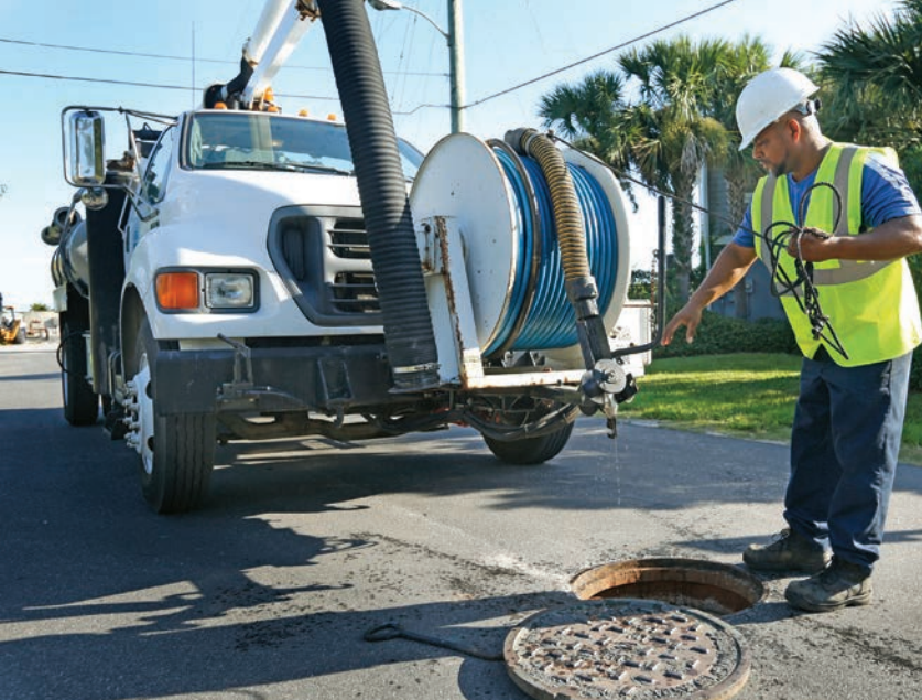
Darrell Noisette wraps up after cleaning a sewer main.
