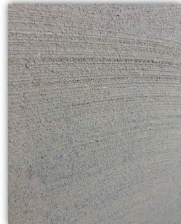
CLOCKWISE, FROM TOP: Properly preparing corroded, contaminated manhole surfaces is critical to ensuring long-term performance of repairs; the finished interior surface of a manhole after mortar application; a coated manhole after full rehabilitation.
