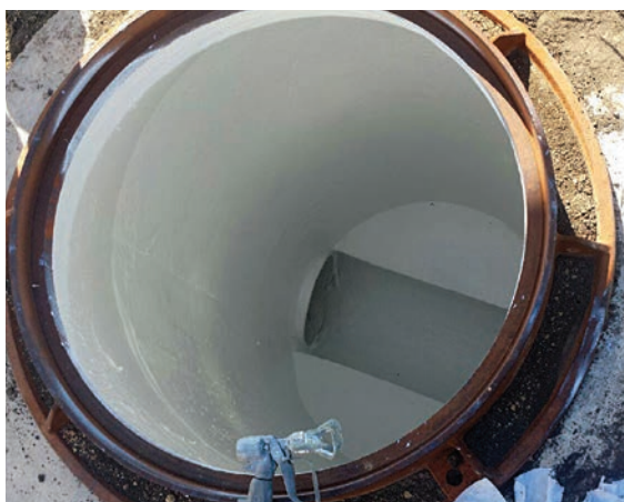
CLOCKWISE, FROM TOP: Properly preparing corroded, contaminated manhole surfaces is critical to ensuring long-term performance of repairs; the finished interior surface of a manhole after mortar application; a coated manhole after full rehabilitation.
