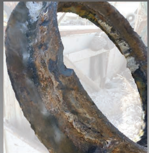
Decaying Frame Walls & Supports
